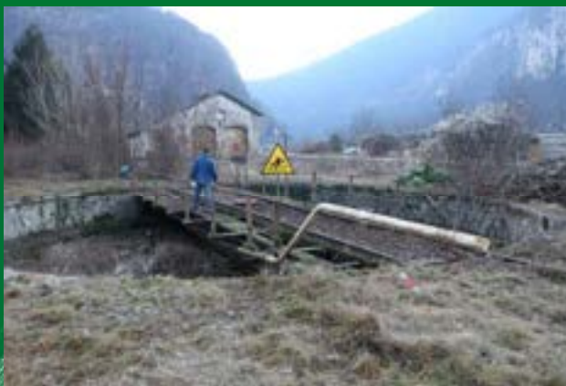
Primolano 2008 – Turntable pit after cleaning
