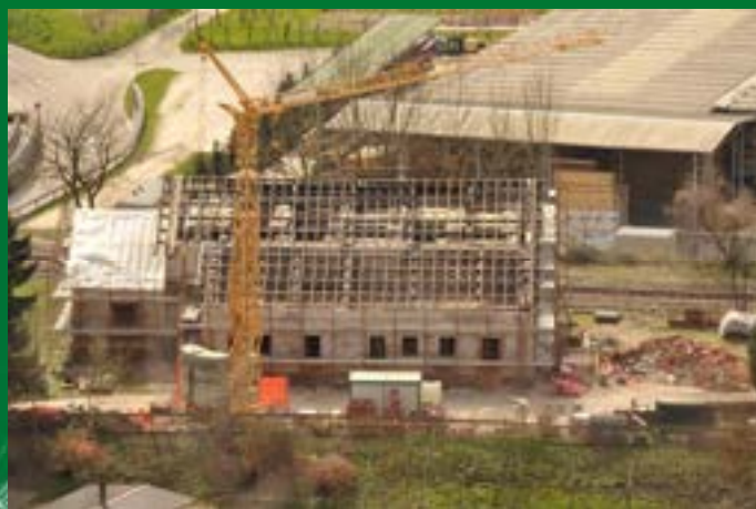
Primolano 2015 – Work in progress on the roof: dismantling is now complete
